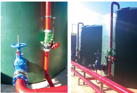
Images: Independent support of the valve (top); Vertically installed tank fill valves (bottom).
