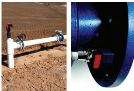
Images: Welcome to the new Bermad Meters website (top). Air valve / mag flow installation out in the field (bottom left); detail of mag flow with pressure sensor in meters (bottom right).
